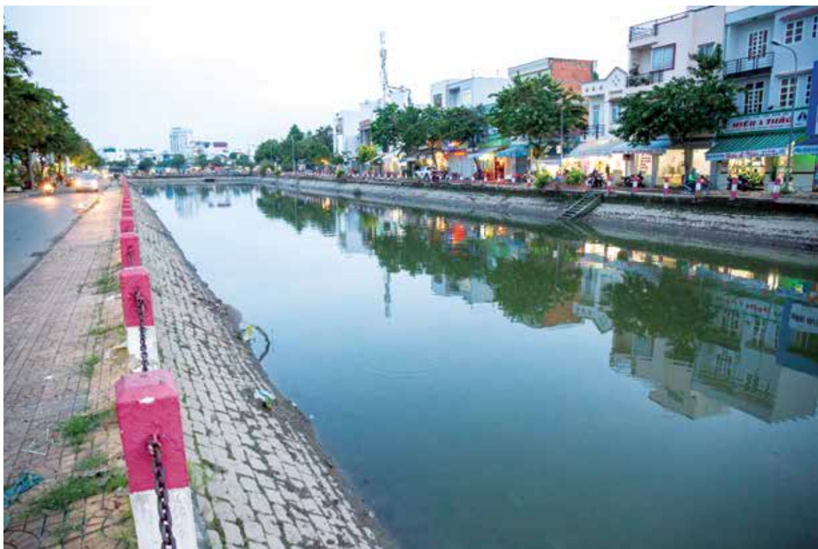
Drainage canal in Can Tho City. Photo © GIZ
