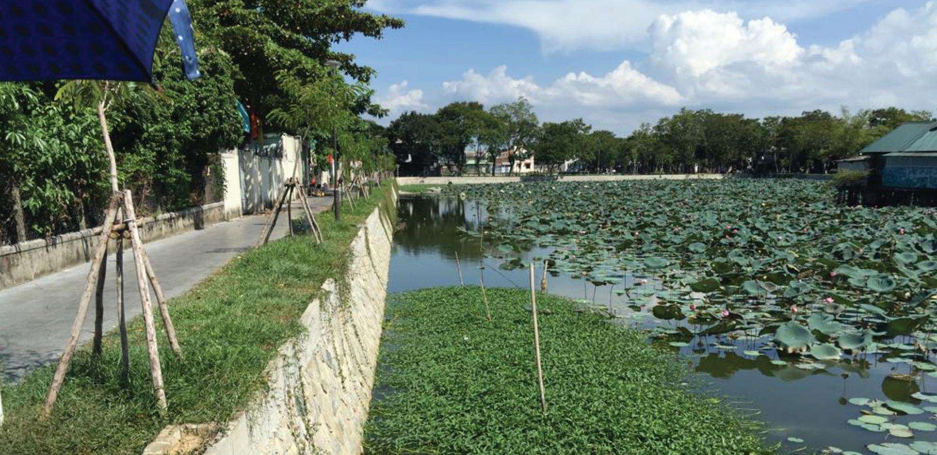
**HUE CITY.** Due to the surrounding hard embankment and years of receiving a mix of stormwater and domestic wastewater, Lap River and ponds in the city suffer from poor water quality. The river has become narrow, inhibiting flow and accumulating heavy sedimentation; the ponds, because of lack of daily water recirculation, are reduced to standing water. The way the embankment is built also discourages people from interacting with the water or natural environment.
