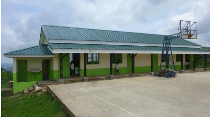
Caption: A newly renovated school building in Mahawan, Kananga, western Leyte. © SDC
