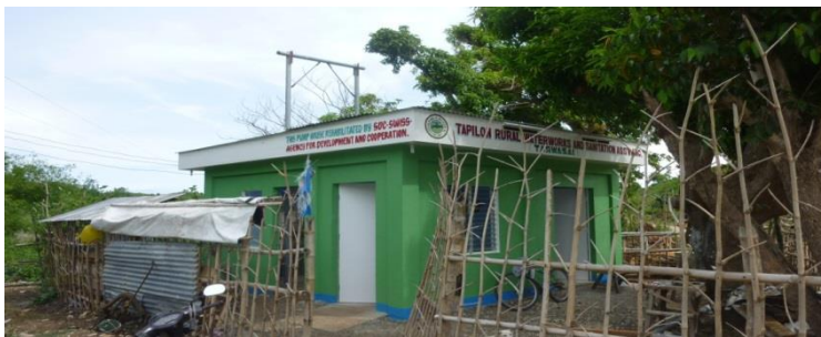
Caption: SHA water experts helped local workers to build a pumping station in Tapilon, northern Cebu. © SDC
