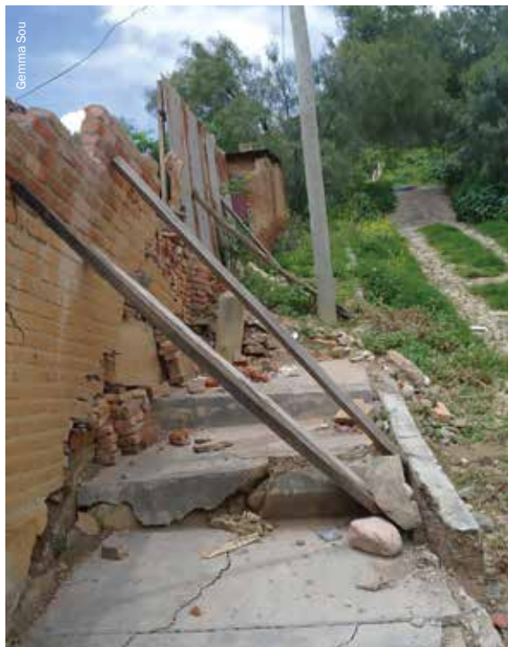
Walls propped up, post-landslide, Cochabamba.
